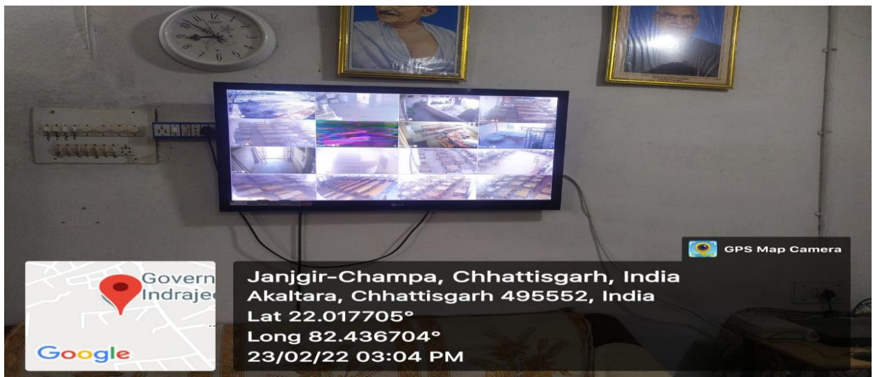
Monitor for CCTV Camera
